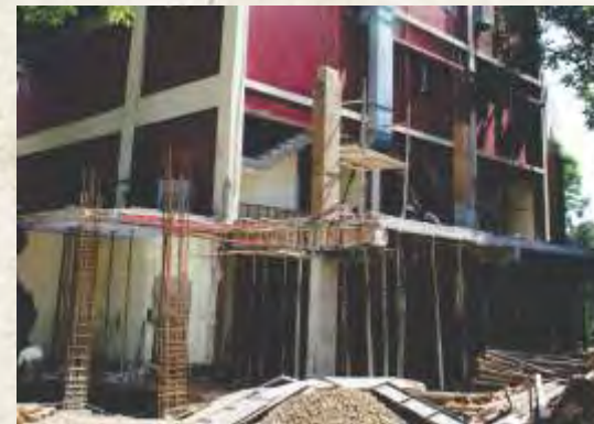
The Boarding House - Work in Progress
